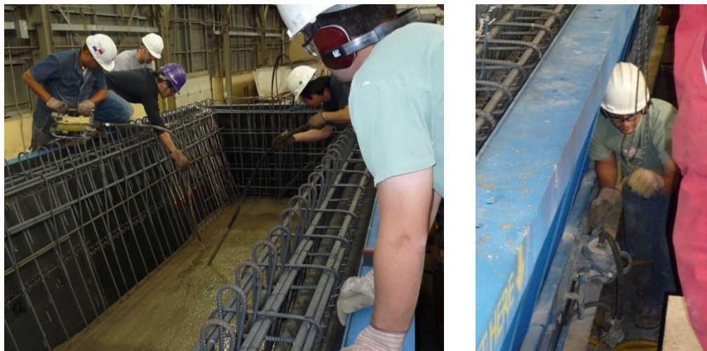
Figure 3.46 Consolidating bottom-flange concrete using internal vibrators & external form vibrators
