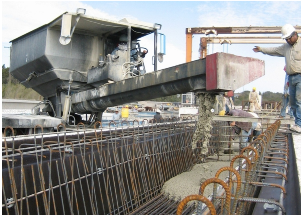
Figure 3.31 Placing concrete using sidewinder (concrete buggy)
