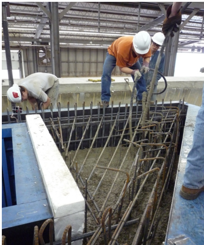
Figure 3.50 Placing concrete in large triangular end block (Beam 2, 45°-skewed end)
