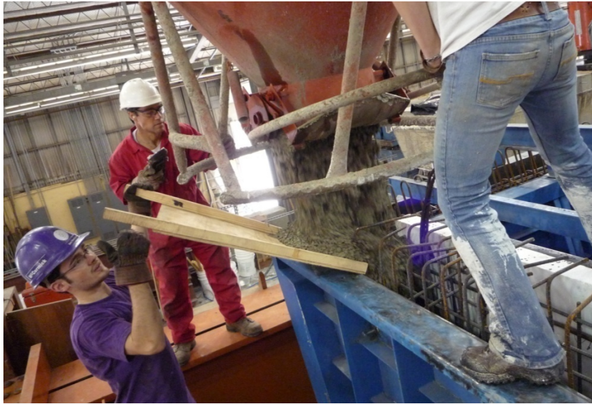
Figure 3.49 Casting end block (and webs) around the interior void
