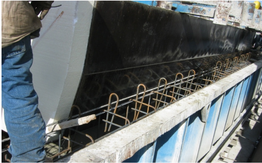
Figure 3.33 Installing the interior-void form
