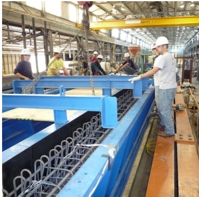
Figure 3.48 Positioning interior-void hangers
