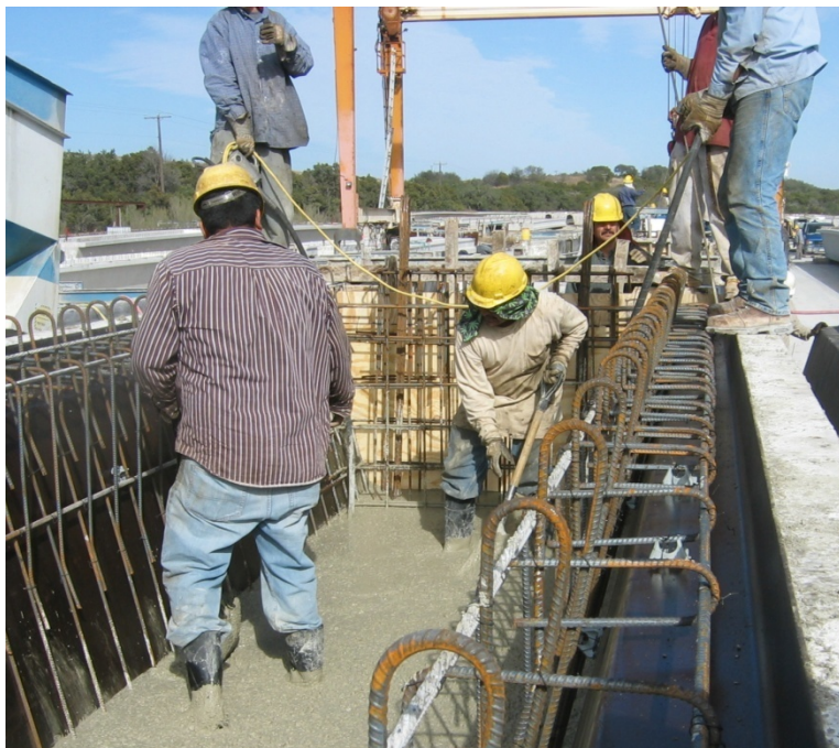
Figure 3.32 Consolidating bottom-flange concrete using internal vibrators & external form vibrators (not shown)
