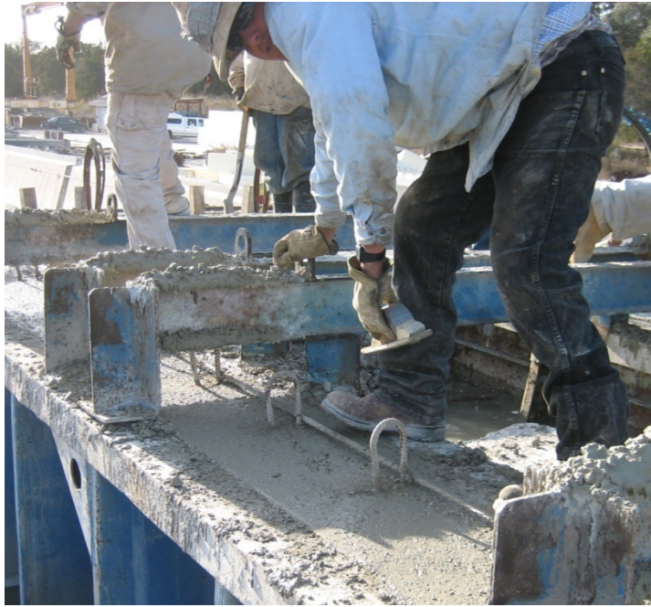
Figure 3.35 Finishing the top surface
