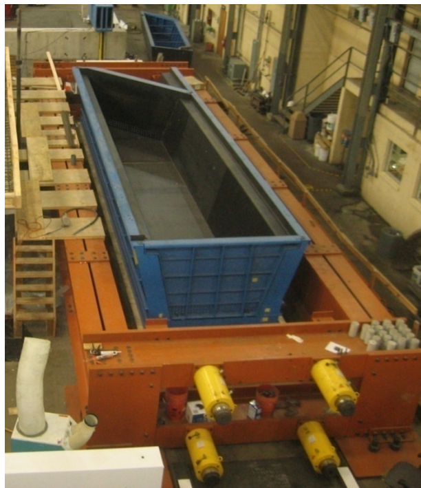
Figure 3.39 U-beam formwork in pretensioning bed
