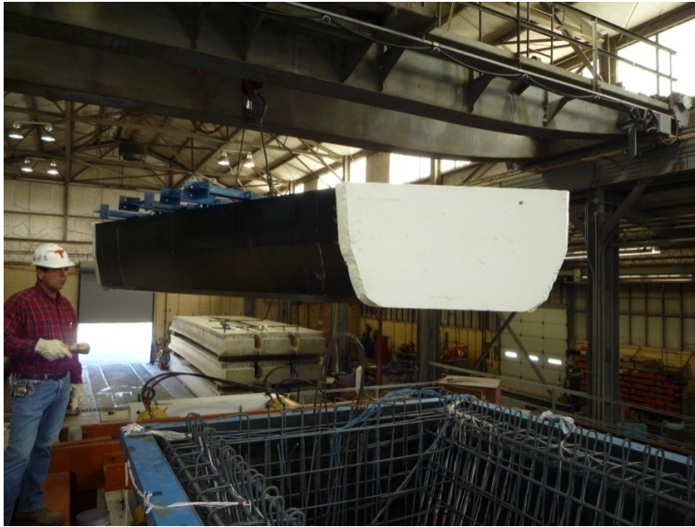
Figure 3.47 Moving interior void into position after bottom flange is cast
