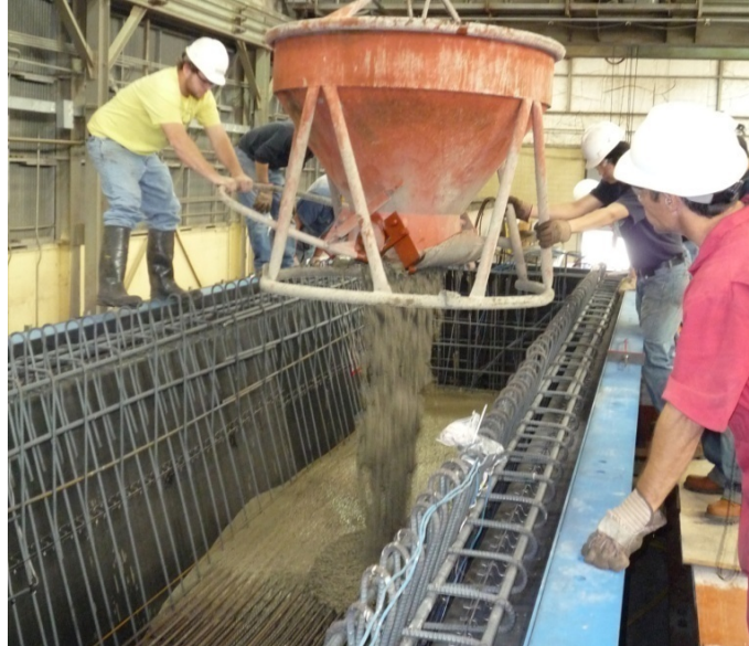
Figure 3.45 Placing concrete in the bottom flange
