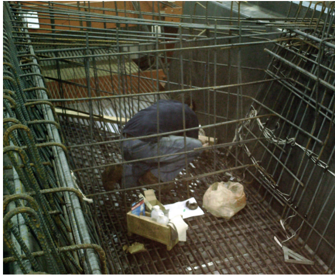
Figure 3.22 Strand strain-gage installation process (Beam 2, 45°-skewed end)
