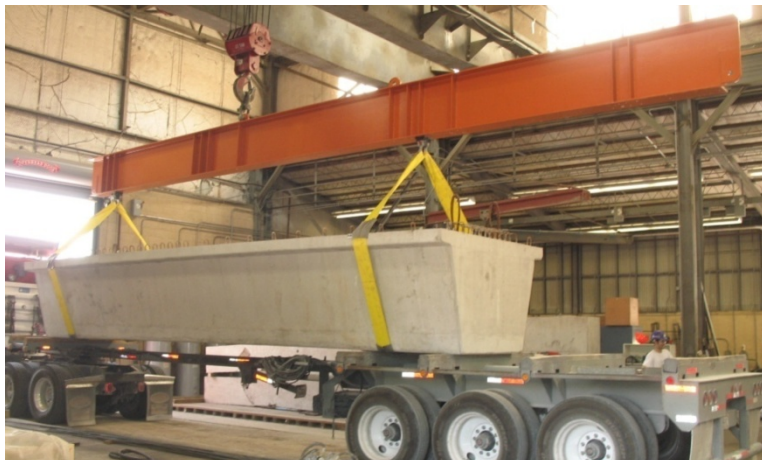
Figure 3.53 Lifting Beam 0 from delivery truck
